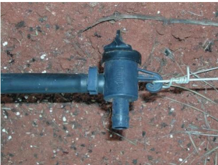
Figure 4. Tap installed on a lateral
