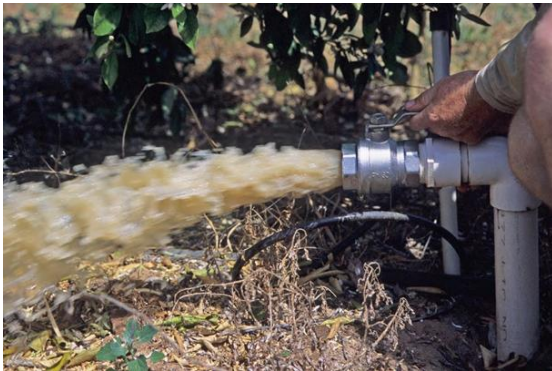
Figure 1. Flushing the submain until water runs clean
