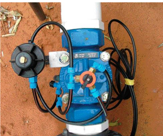
Figure 6. Three-way hydraulic valve
